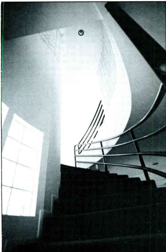
Figure 7. This glass-block enclosed stair goes from ground level to the studio.
