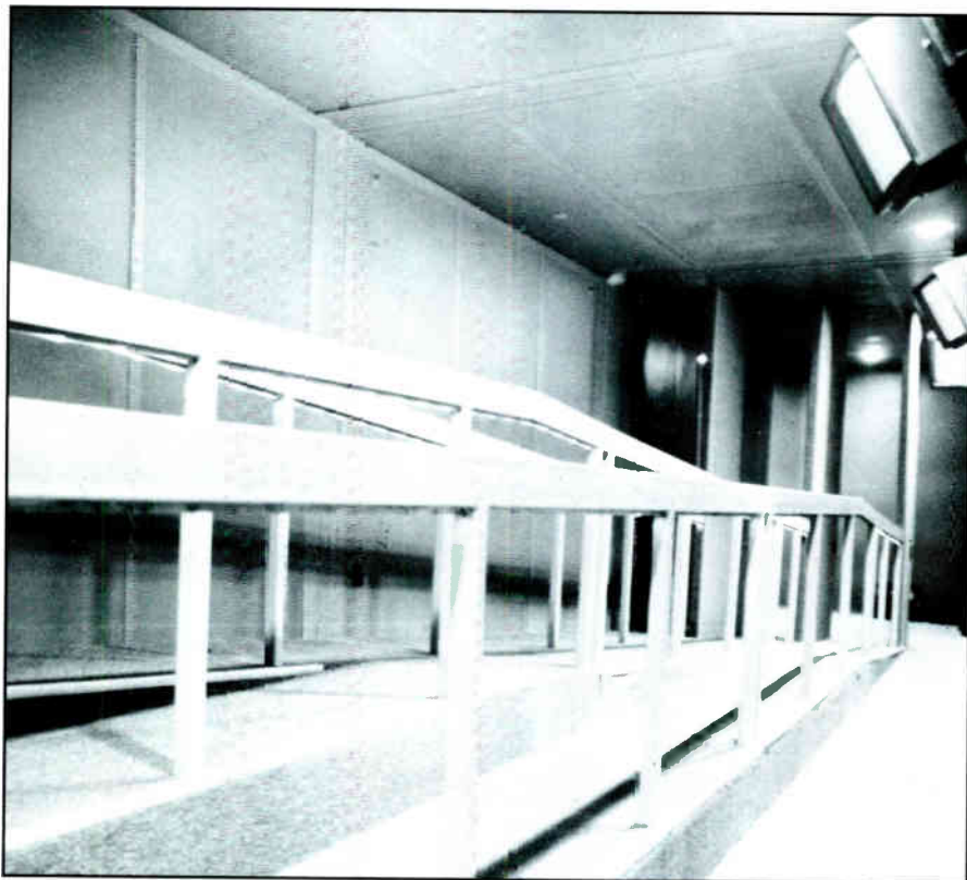
Figure 2. IAC Moduline System components (note back wall) are only 4-inches thick yet provide the sound conditioning required. The light weight facilitates relocation of the Viewing Tube.
