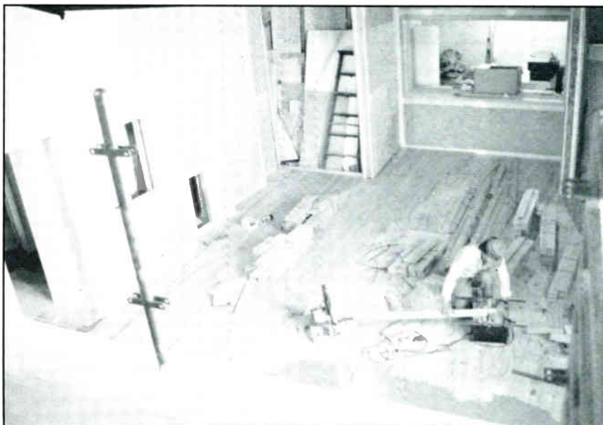
Figure 3. A detail of the interior framing in the studio room.
