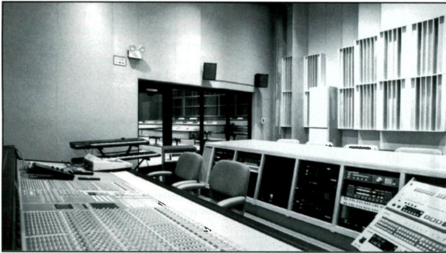
Figure 3. Control Room A looking across the SSL 4000G Series console and beyond into the classroom lab.
