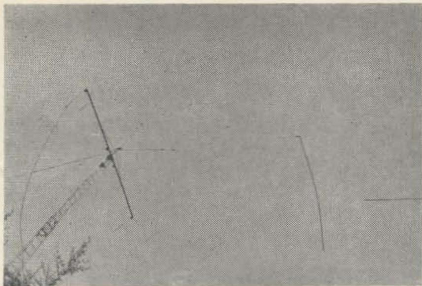
2 element 40 meter wire beam shown with ground plane. Note the long spring at right to compensate for tree movement in wind. The ground plane has been replaced with a two element rotary.
