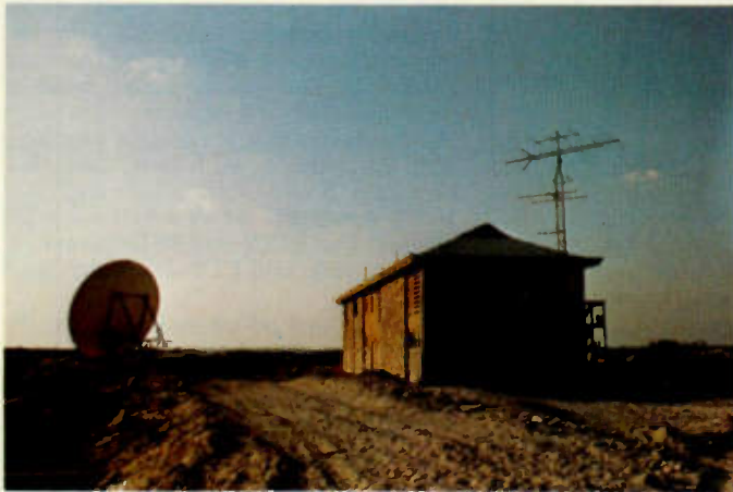
The dish and studio building of WIV. The antennas pick up TV from Miami during openings. They also send the satellite signals via channel 7 to a hilltop, where a solar-powered transmitter rebroadcasts on channel 4 for the whole island. It's free for now, but Bob intends to encode the signals and charge . . . much like cable TV.
