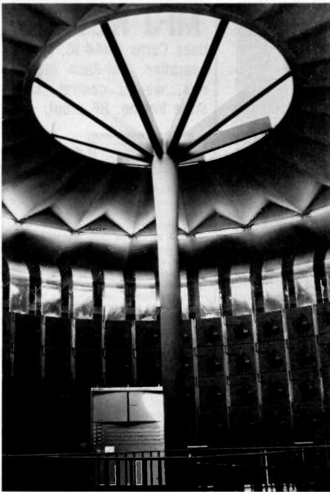
*Antenna side-switching hut showing a portion of antenna routing system. Each "square" is a motor-driven switch.*
