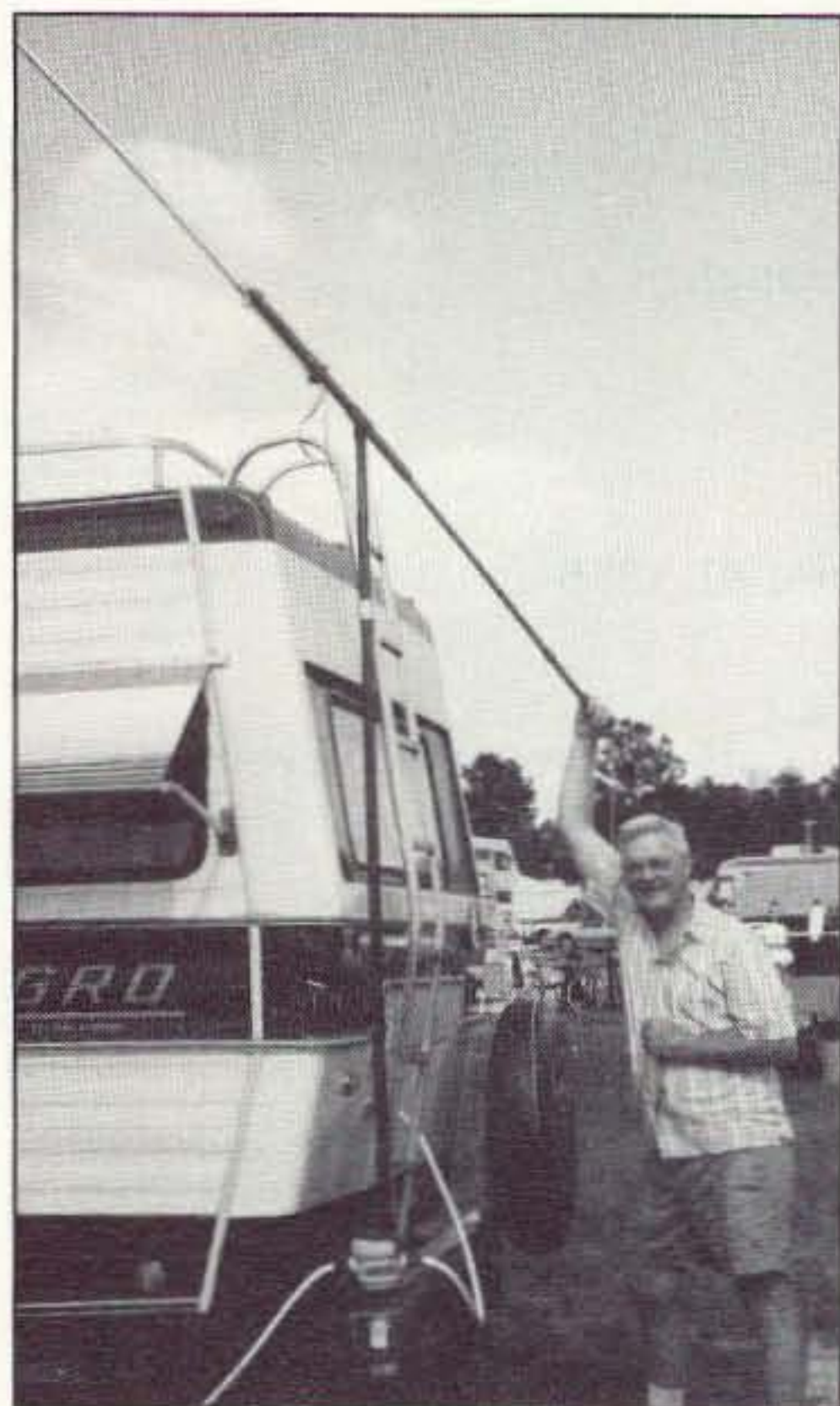
Photo D. Pull the 1/2" pipe all the way out with the rope, then pull down to raise the antenna. Tie off the rope to secure.
