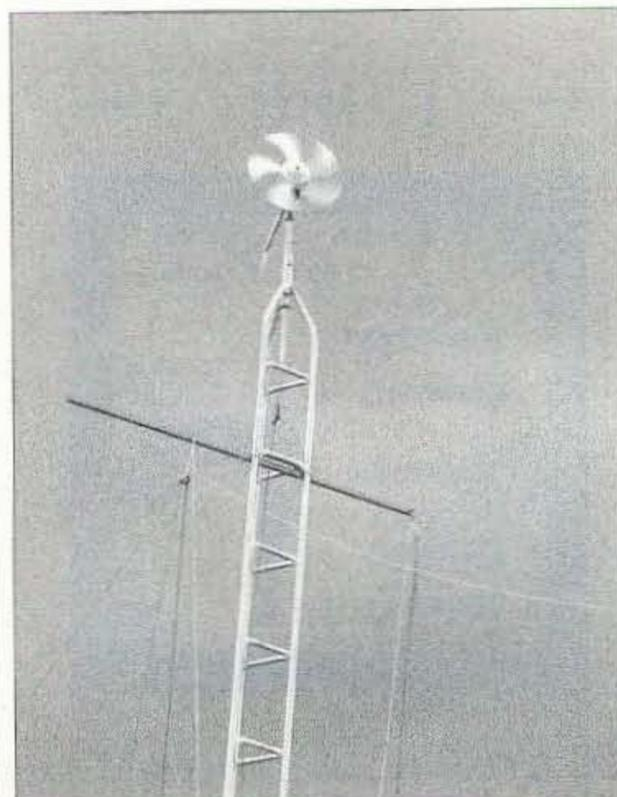
**Photo H.** High atop the tower, the Microwind generator charges the station batteries as storm clouds gather in the background. The tiny machine can survive and produce power in storms that would destroy a larger wind generator.
