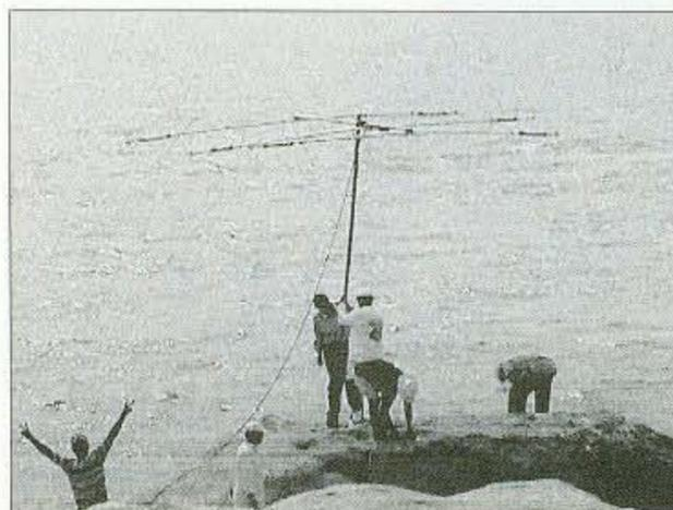
**Photo L.** MA5B Cushcraft antenna being installed. This was the antenna for Station 1. The mast and guys were fixed to the rock by anchor bolts drilled into the granite. It stood well for the entire two windy days.
