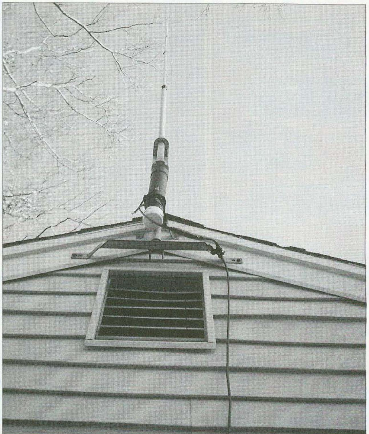
Photo A. This meager antenna is capable of operating on 160 and 80 meters.
