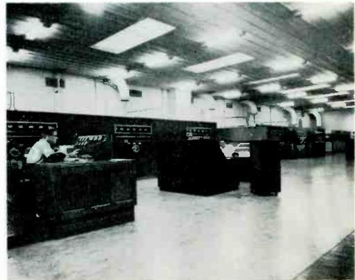
Radio Australia's Transmitter Hall at Shepparton, Victoria. Incoming programs from Melbourne for VLA, VLB, and VLC transmitters are controlled by a technician at the master panel (left).
