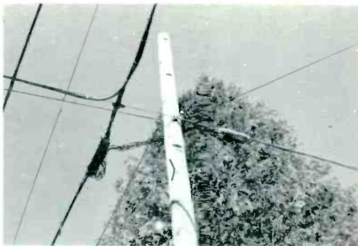
**AND AFTER!** Twin lead gone. Power transformer gone. Line amplifier boxes gone! *But, same pole.* Now all line amplifiers mount at the base of the poles, and 110 volts is "on the ground" as prescribed by law. Coax feeds the system, in place of the seven-year-old flat line.
