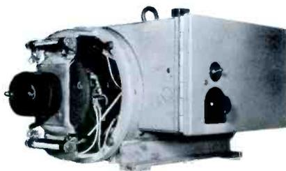
The unit has a 2 HP, 220 volt DC motor driving a 1 KW, single phase, 115 volt, 60 cycle generator. Operating speed
