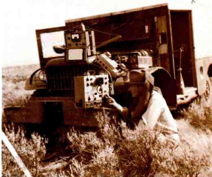
Walt Szemanski, on a mountain top at Richland, Washington, using a marker generator to locate an interfering radar signal.
