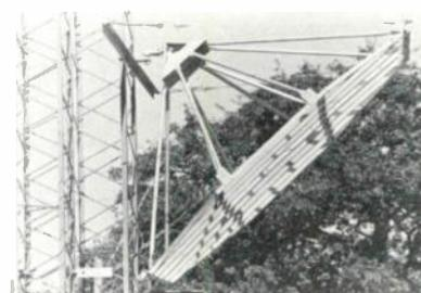
The most simplified design ever developed for CATV! This precision-made unit is your answer to microwave reflector problems. Octagonal shape is composed of two interchangeable halves for easy assembly and maintenance. May be converted into a paraboloid by the simple turn of a screw. Check these other outstanding features:
