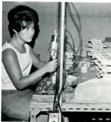
Final assembly of directional taps includes putting self-tapping screws in the lid, and installing the tap legs and terminators on the base of the unit.
