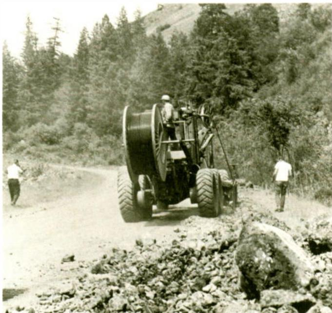
Flexibility and durability are necessary characteristics of direct buried cable. Shown above and in the photo on page 103 is Anaconda Sealmetic going underground.
