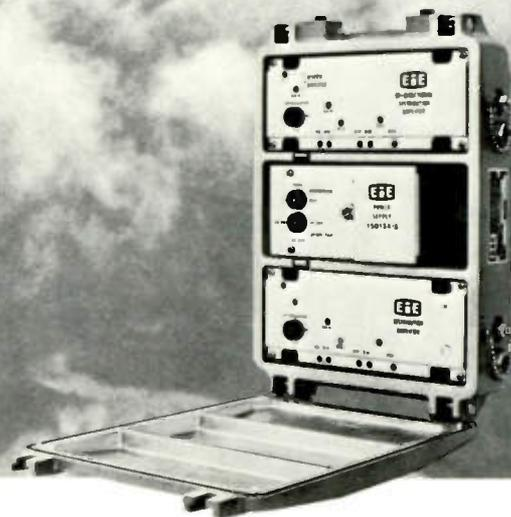
... and it's happening now with EiE Two-Way. A complete system capability that is compatible for new construction or readily inter-faced with your existing cable system. Everything from the head-end to subscriber's set, including a rugged line of trunk, bridger-trunk, distribution amplifiers, modulators and a new shielded, coaxial A/B switch.
