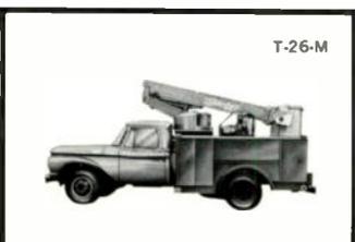
Long 26' reach on small vehicle. Easy bucket access. Built-in electric power. Capacity 300 lbs. for transfer and reconstruction.
