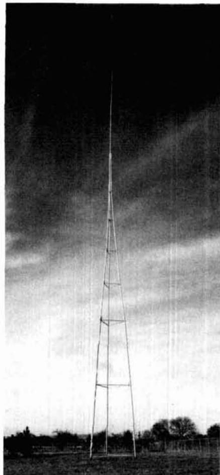
fig. 8. The self-supporting 160/80-meter vertical antenna at K6KBE.
