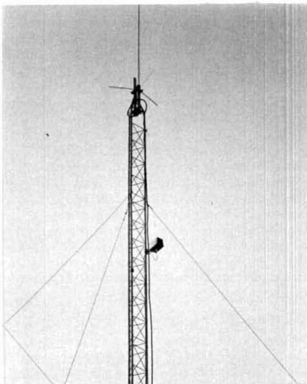
fig. 8. X-band beacon is perched near top of tower.
