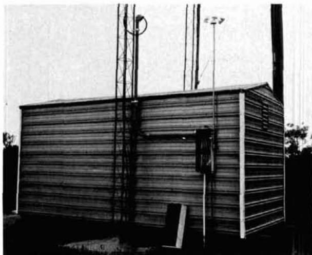
fig. 10. Coax enters building through a weather-proof box. The anemometer is made from a DC motor and recycled air freshener containers.
