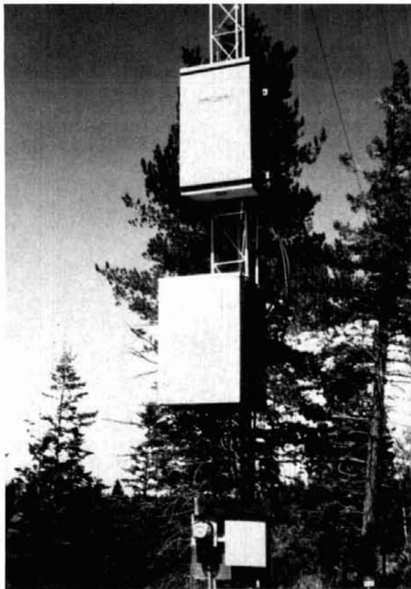
**Photo B.** Waterproof boxes near the base of the Zia Connection tower at Benson Ridge, New Mexico house all equipment.
