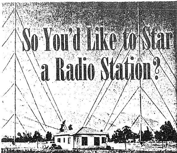
TRANSMITTER HOUSE in the Pasadena Valley. Great difficulty was experienced in getting this piece of property; Japanese squatters had planted the land in strawberries and refused to get off.
