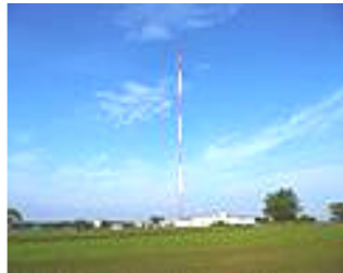
JOGB Transmitter Site
