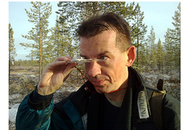
Mika checking the direction while carrying the cable reel of the 30 degree antenna
