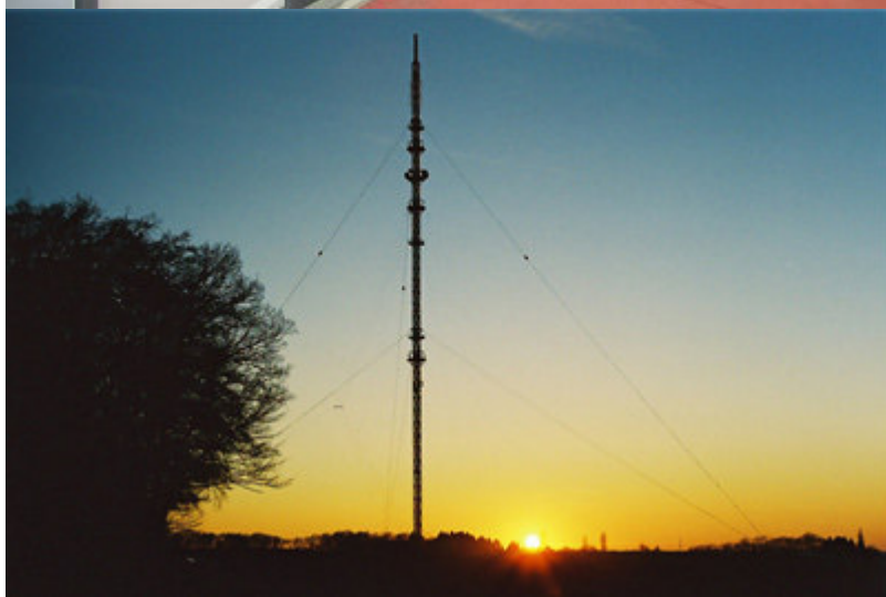
Antenna "Hordt" (301m)
