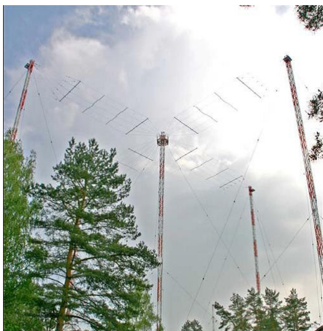
← Horizontal cross dipole antenna for MW broadcasting in Mainflingen
