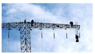
A face lift [see photo] will remove the top structures that were added to the towers in 1954. This will reduce the wind load significantly and give the masts their original 1927 "slim-line" look back. Only the inner two of the eight top capacitance wires that also feed the secondary tower of the Alexanderson antenna system will be retained.
