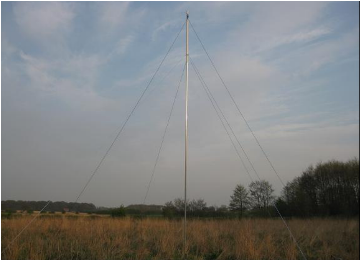
Figure 1: One of the masts showing the four guy ropes and the antenna loop at the very top of the mast.
