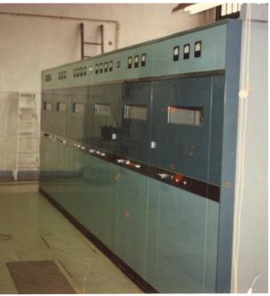
stations that once existed in the USA... (the) MRHS felt it needed its own coast station to carry on the traditions and preserve the skills of the art of maritime radio through actual use. KSM uses the original transmitters, receivers and antennas of KPH. The station is licensed for communications with ships at sea using both CW and RTTY modes in the MF and HF marine bands. KSM accepts traffic from ships at sea for onward transmission to addressees ashore. No charge is made for this service."
