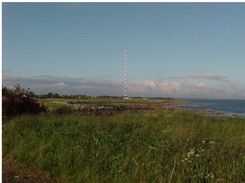
Kvitsøy site. It is still the operational centre for Norkring's
