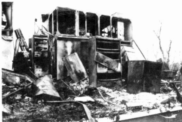
A view of what was left of a transmitter.
