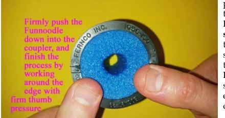
plumbing coupler, using firm downward thumb pressure on alternating sections of the Funnoodle, until it reaches the position **shown in the photo**. Check the other edge of the plumbing coupler to ensure that it has a similar appearance, and if not, use firm thumb pressure on either side of the Funnoodle until both of its sides have a similar flat appearance. Ensure that neither edge of the Funnodle extends past the edge of the plumbing coupler.
