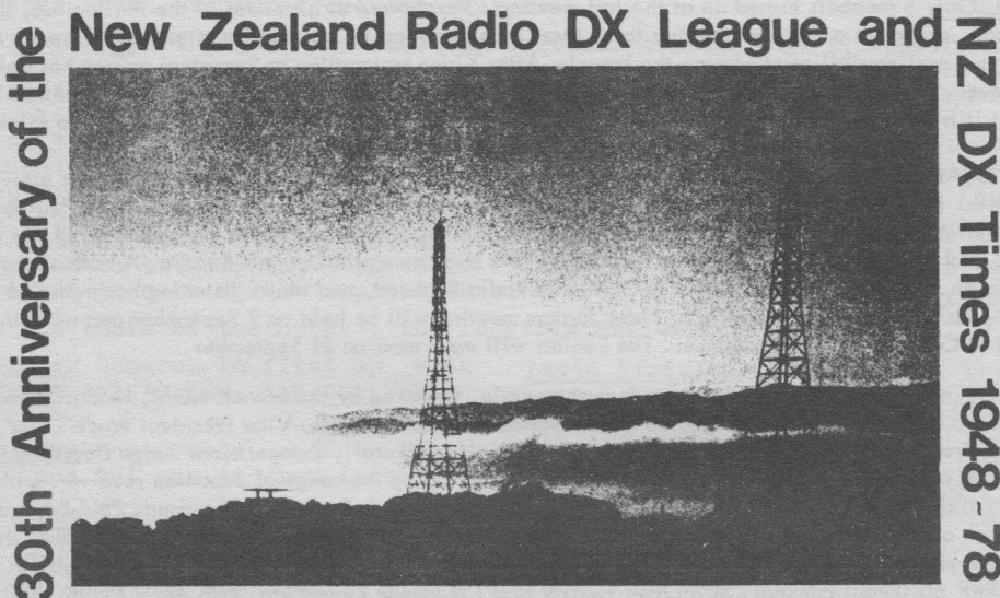
Early morning fog enshrouds the antenna towers of Radio 2ZM 1130kHz, atop Mount Victoria, Wellington. (photo courtesy 'Evening Post')
