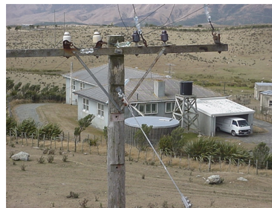
View of Quartz Hill Receiving Station at Makara near Wellington. For more information on using the Quartz Hill facilities at Makara near Wellington. Contact Mark Nicholls 4 Parera Grove , Heretaunga , Upper Hutt 6007 phone 04 972 2606 or 021 376058 email mark@radiodx.com
