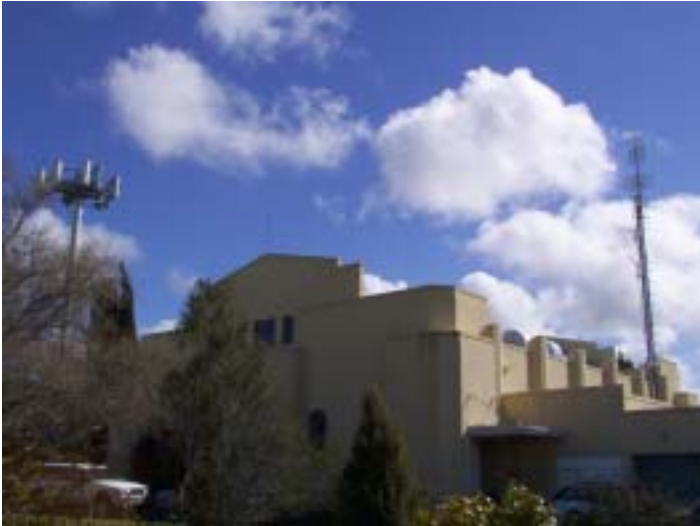
The building which houses 11 transmitters
