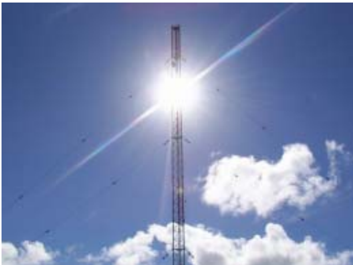
Transmitter Mast out the Back
