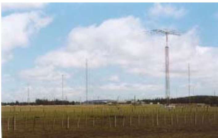
Log periodic and rhombic antennas just north of Waiouru. September 2001 Photo credit. Bryan Clark
