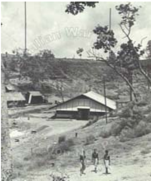
General view of the 9PA studio and buildings with the 90 foot aerial masts nearing completion on the ridge in the background. Photo taken on February 14, 1944. Australian War Memorial (c).
