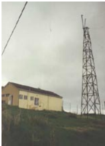
The North wing of Radio St. Helena showing one of two Aerial Towers © Copyright Radio St. Helena
