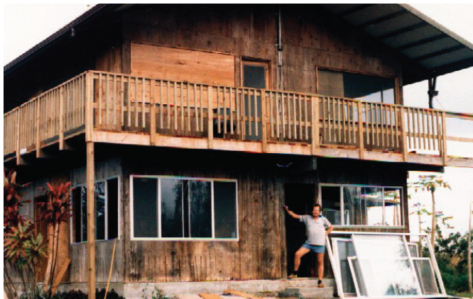
Richard Woods partly completed house.
