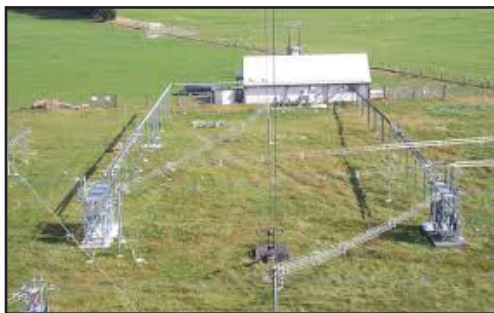
Part of the RNZI transmitter site at Rangitaiki (c/o radionz.co.nz)
