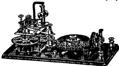
THE OMNIGRAPH AUTOMATIC TRANSMITTER, connected with sounder, or Buzzer, will send you unlimited Continental or Morse Code messages, at any speed you desire.
