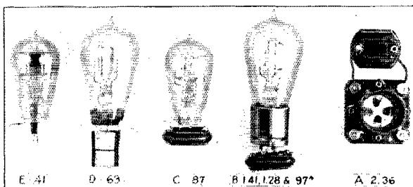
GROUP OF SHORT-WAVE ULTRAUDION OSCILLATORS SHOWING CONSTRUCTION NEEDED WHEN OPERATING AT  $\frac{3}{4}$  M. DIRECTLY AND ADVANTAGE OF WORKING IN MANNER SUGGESTED. THIS IS THE GROUP MENTIONED BEFORE AS USED BY PHELPS AT 2EB.
