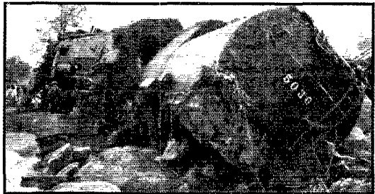
ONE OF THE LOCOMOTIVES BURIED IN THE SILT OF CALIENTE CREEK BED DURING THE RECENT CALIFORNIA FLOOD
