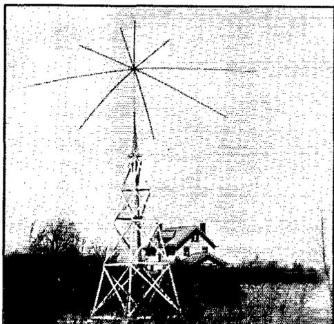
A RIGID TOWER EQUIPPED WITH A ROTATING MECHANISM SUPPORTS THE WEB ASSEMBLY AT W8MJM
