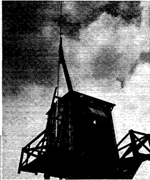
A close-up of one of the 20-foot dipoles of the Adcock direction finder. Adjustment of this antenna is so critical that even a spider-web across the transmission line will cause an error in taking a bearing.
