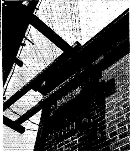
Above — The terminal point for the directional antennas that are located several miles from the main station. They connect to a selector switch in the cruising room. Upon hearing a signal the operator can then determine the general direction of the transmitter.
