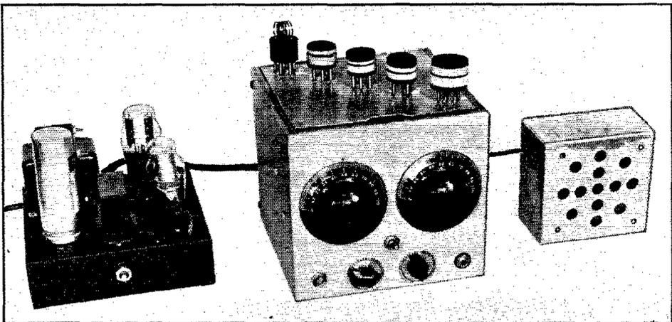
The beginner's receiver, complete with power supply, cabinet, coils and loudspeaker. The stand-by switch is at the lower left on the receiver panel. Regeneration and volume controls are in the center at the bottom, with the heater-filament switch centered above them. The 'phone jack is at the extreme right. Both main and bandspread tuning dials are of the vernier type.
