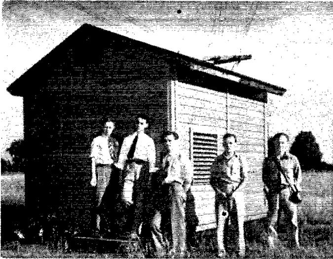
Above—A small frame building houses the three RCA 200-watt remotely controlled transmitters and the Onan 5-kw. emergency gasoline-driven a.c. generator. Folded dipoles and miscellaneous doublets are supported by three telephone poles. Left—Irl Ball, W8VNY; Ken Miller, W5AOC; Bill Hoffert, W5HVB; Dick Boll, W9EVD and the watchman pause to have their picture taken in front of the transmitter house.
