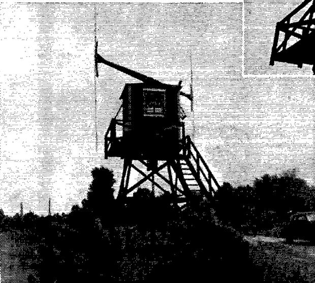
Three folded dipoles are supported in a V-shaped pattern around and above the transmitter house. Telephone poles are spread out in every direction like trees in a huge forest. We found that they lead to eight rhombic antennas which are oriented to cover 360 degrees. In addition there are three Beverage antennas, a dozen folded dipoles, miscellaneous ultrahigh-frequency doublets and a special array of transmitting dipoles near the transmitter house.
