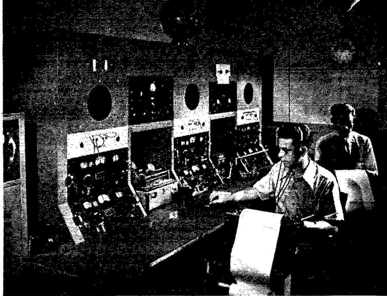
*Below*— Transmissions being recorded on Memorex discs. Each drawer beneath the amplifier includes a turntable and a magnetic recording head which embosses on paper based discs one hour and five minutes of playing time per side. The operator here is transcribing signals which have been previously recorded.
