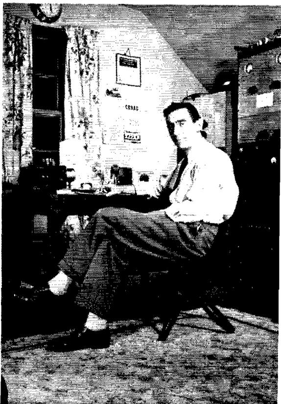
It isn't easy to score a "first" these days, but John Erhart, W2TGO, managed the trick when he worked DL4PA for the first amateur two-way single-sideband trans-Atlantic contact. The rig is a crystal-filter job starting at 80 kc. and ending up with a pair of HK-257Bs in Class AB<sub>1</sub> running about 400 watts peak. The antenna is a 14-Mc. W8JK.
