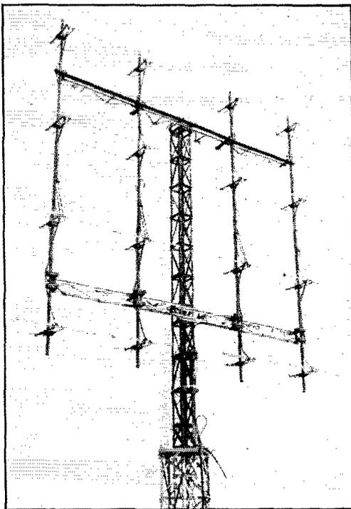
The City Slicker's country cousin — the 32-element array of W8WJC, Everet, Ohio. Four City Slickers backed up by reflectors tower 95 feet above the highest spot in Summit County.
