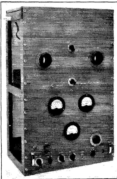
Front view of the completed transmitter. The 6L6 input tuning control, crystal-VFO switch, 6L6 output tuning control, 807 input control, 807 filament switch ( $S_2$ ), meter switch and key jack are equally spaced along the bottom edge of the exciter panel. The VFO input connector and crystal socket are above to the left and the 807 output tank-condenser control to the right.
