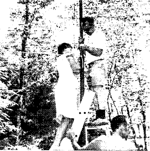
WA3ATQ assisting, OMs W3KKN holding the mast, W3QXT steadying the ladder, installing FD antennas for PJ-YL.
