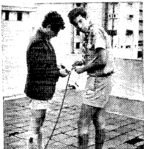
▲ Atop a ten-story building, Scouts string up antennas for CR71A in Mozambique.
