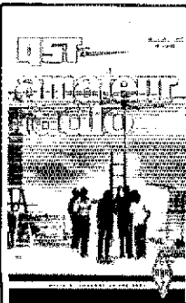
OUR COVER Installing the 20 meter beam at the W6VB/6 FD site. Complete FD results start on page 56.
