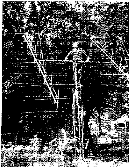
WA4GPM adjusts the position of his 80-element collinear for 2-meter EME.
