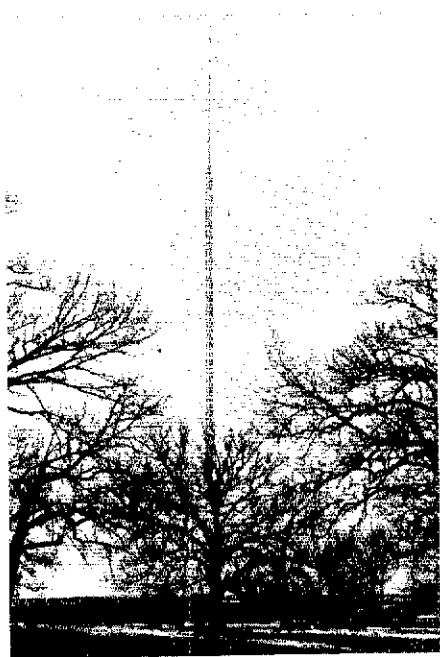
The major noise source at W9UCW is the 160-meter vertical (Minooka Special).
