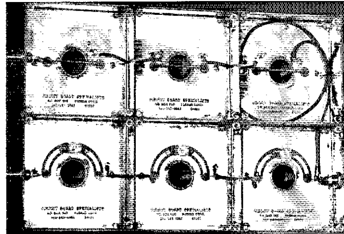
Fig. 12 — This photograph shows the interconnecting wires used between the six cavities in the duplexer. All shielded cables are RG-174/U. At the far right is the 17-inch length of cable used to connect the low-pass section to the antenna connector.
